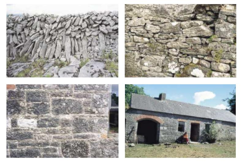
A range of stone wall constructions and building materials: left upper, dry-stone walling; right upper, rubble stone construction; left lower, snecked limestone wall; right lower, Liscannor slates on roof. The patterns and textures created by different forms of masonry help to define the character of a building and landscape and can be recognised by the child.
