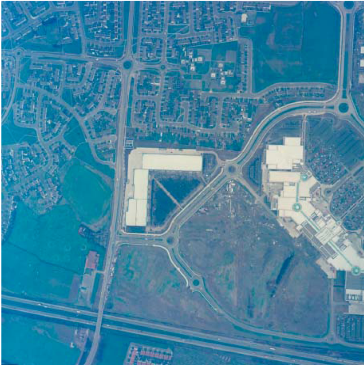
AERIAL PHOTOGRAPH, LIFFEY VALLEY RETAIL PARK
